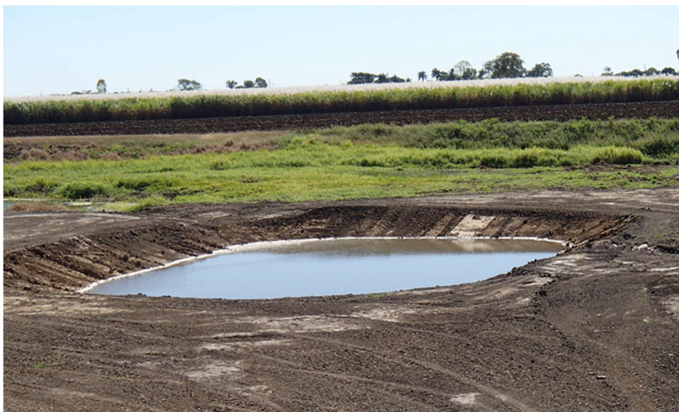
Figure 7: Top: Diagram to show how a sediment basin captures run-off water. Bottom: A newly constructed sediment basin (Source WetlandInfo 2018c).
